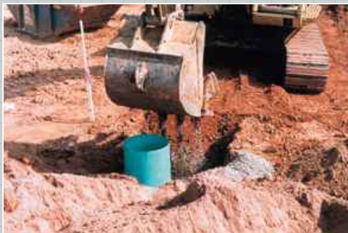
6 Backfill evenly around Drain Basin with stone and compact.
