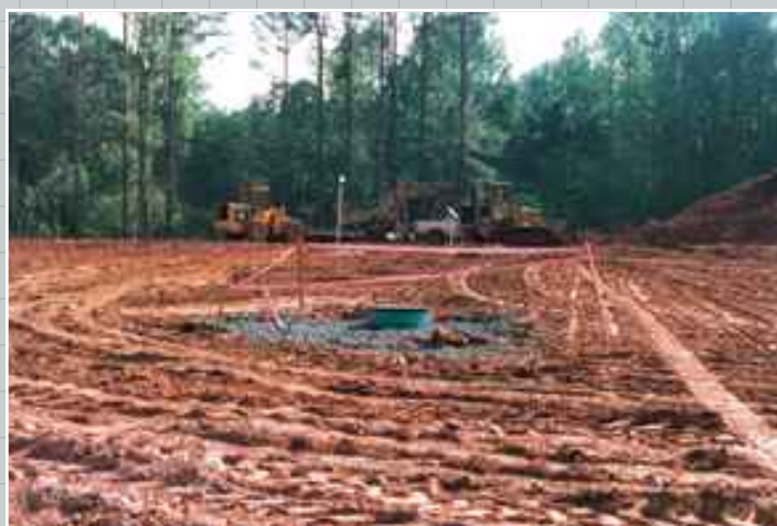
7 Cut PVC Drain Basin body to final grade elevation. If setting Drain Basin and grate for H-20 load, pour concrete ring underneath the grate frame as per installation instructions on Nyloplast CD.
