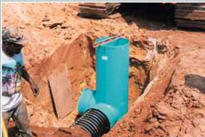
5 Re-check Drain Basin depth, level and position
